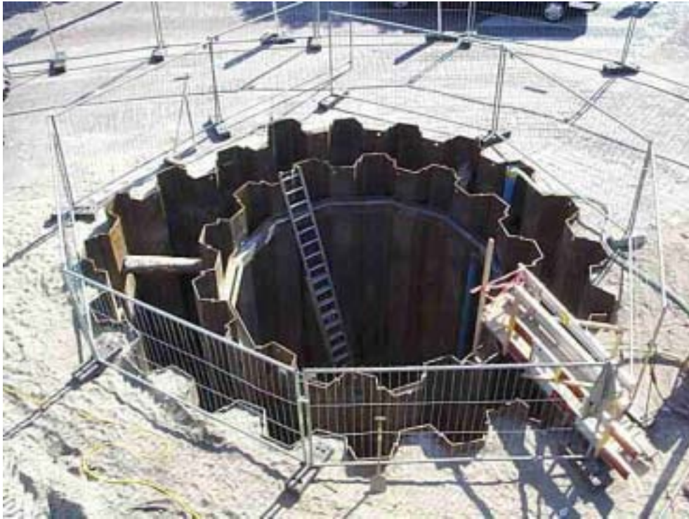
Fig. 8. Gate construction at the test site.
